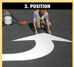
Position the PreMark® material according to layout.
