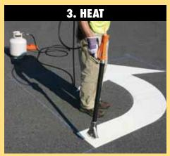
Heat the PreMark® with a propane heat torch such as the Flint 2000EX Heat Torch then chisel test to ensure proper bond.
